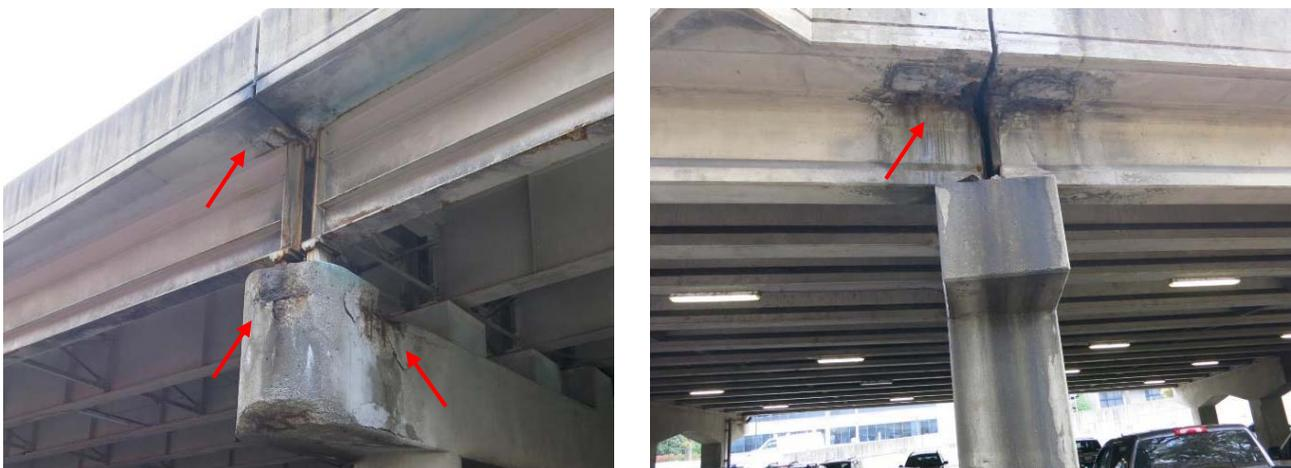
Figure ES5: Typical Pier Joint Leakage and Concrete Damage
