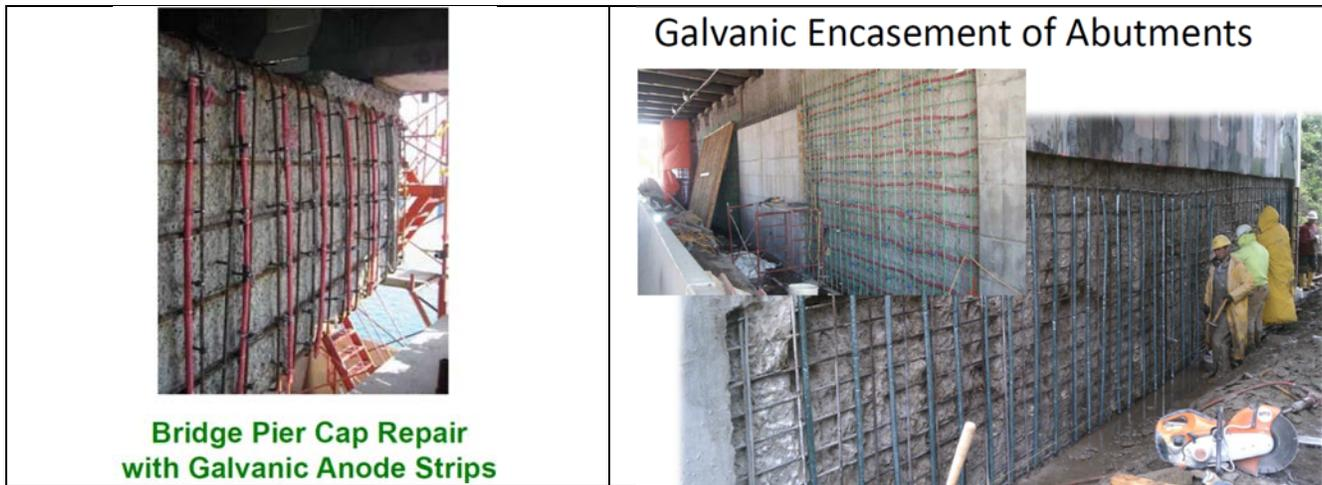
Figure 18: Substructure Repairs with Galvanic Anodes (Vector Corrosion Technologies presentation)
