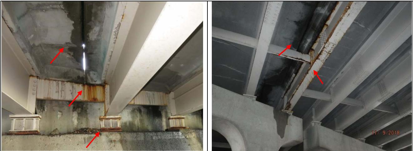
Figure 15: Typical Median Joint Leakage and Corrosion
