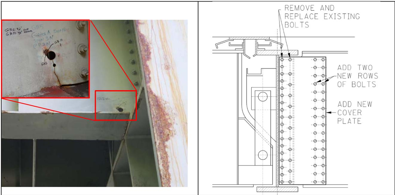
Figure 23: Steel Girder Crack and Cover Plate Repair Option
