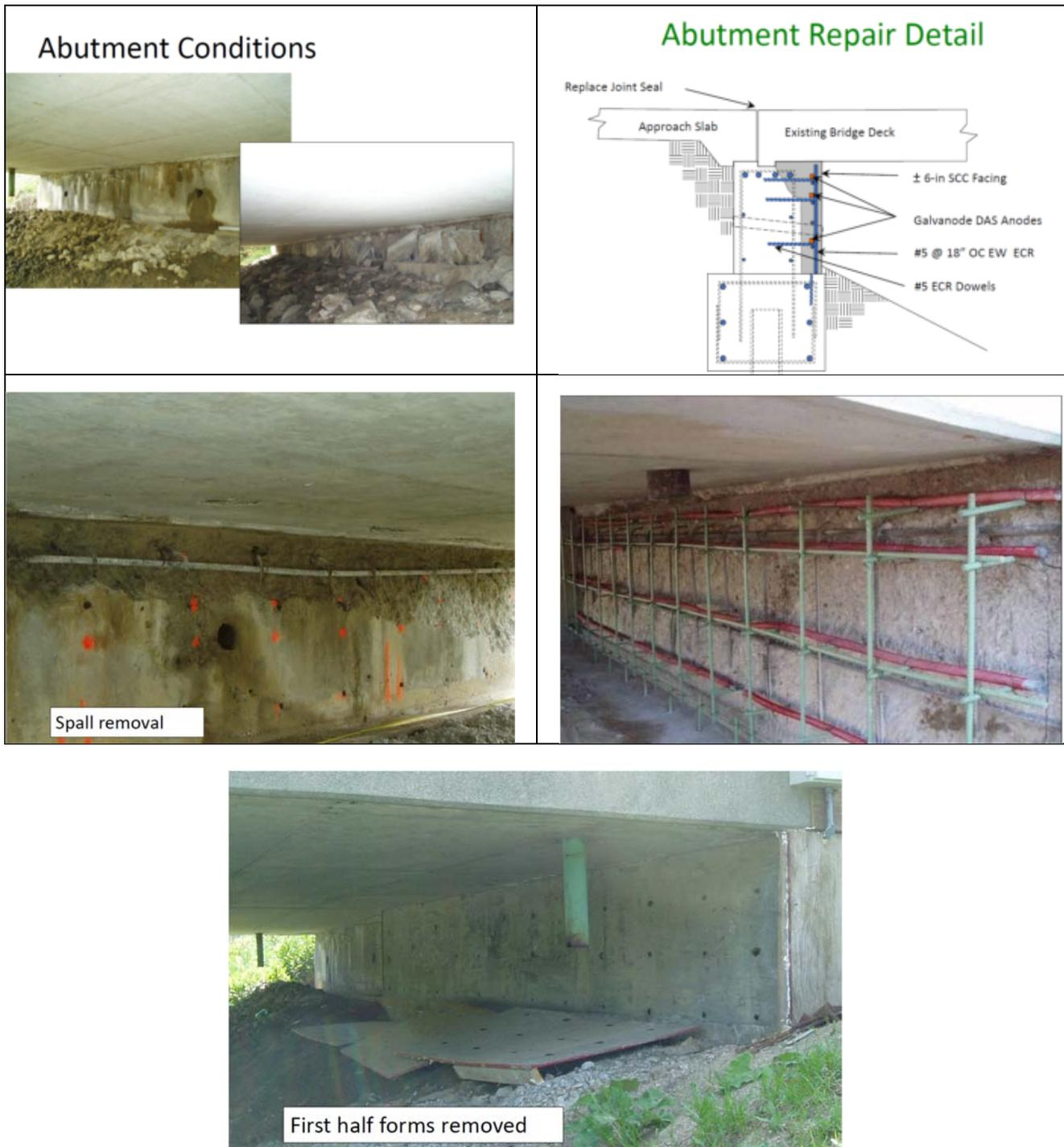
Figure 17: Abutment Repairs with Cathodic Protection (Vector Corrosion Technologies presentation)
