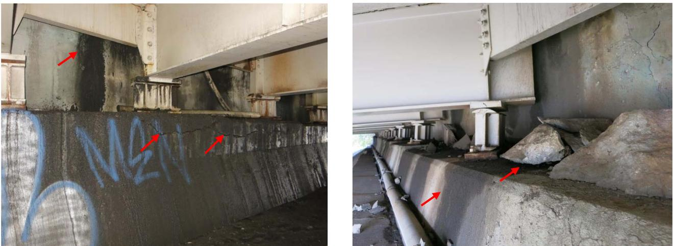
Figure 9a: Typical Abutment Joint Leakage and Concrete Damage
