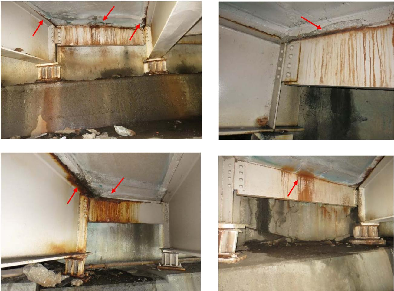
Figure 12: Typical Slab Delamination at Bridge Ends
