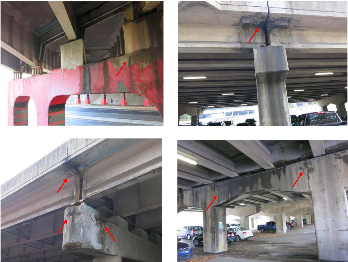
Figure 13: Typical Pier Joint Leakage and Concrete Damage
