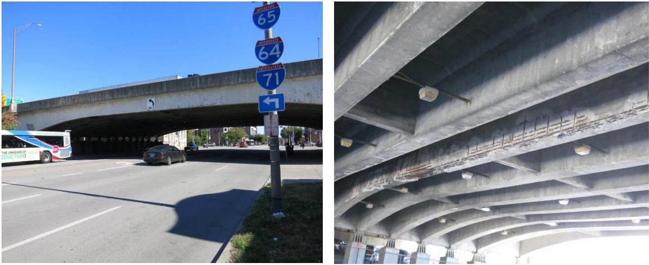
Figure 27: Bridge 191N over Broadway Street showing Corroded Concrete Girder
