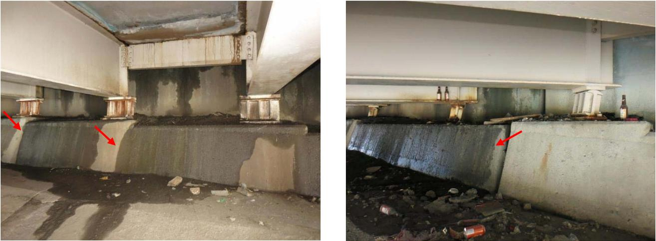
Figure 9b: Typical Abutment Joint Leakage and Concrete Damage
