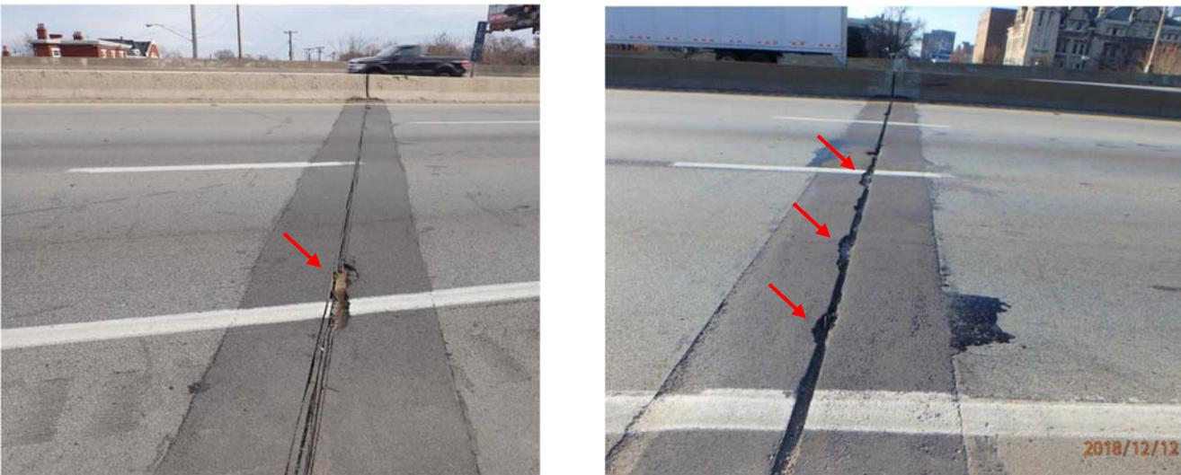
Figure 10: Expansion Joints Replaced in 2017 showing signs of distress in 2018 Inspections
